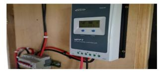
Gambar 2.11 Solar Charge Controller
