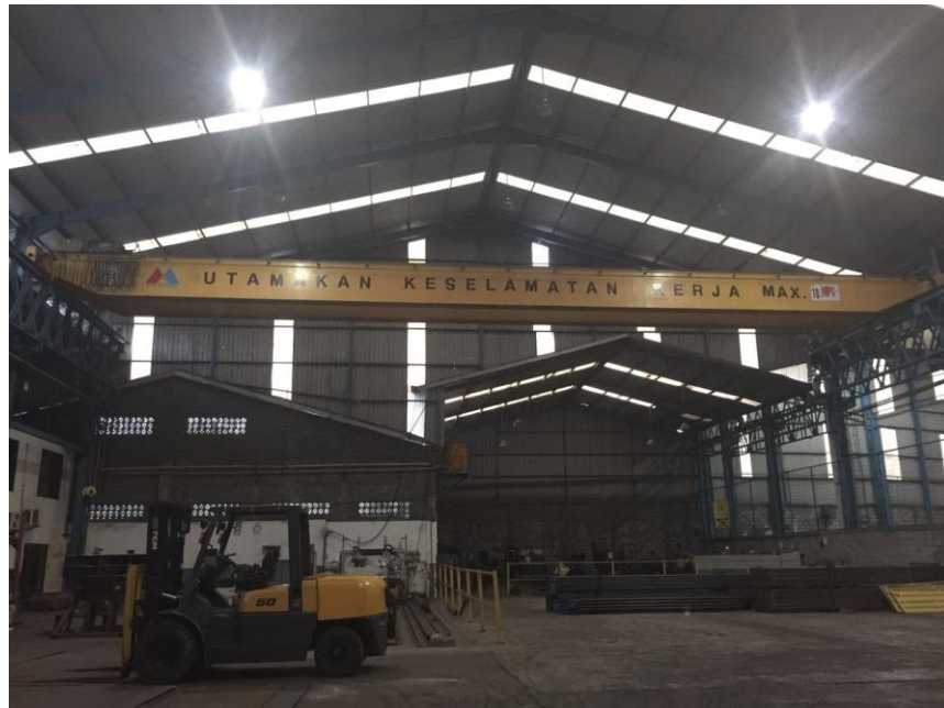
Figure 1.1 Hoist crane at Mitra Adyaniaga.PT, the manufacture of boilers, Surabaya - Indonesia
